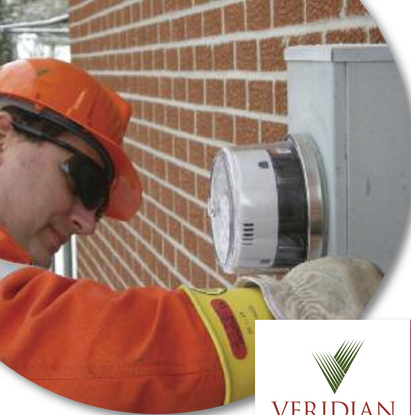
Veridian's Aaron Goldman installs a residential smart meter. (Photo courtesy of Veridian Connections)
