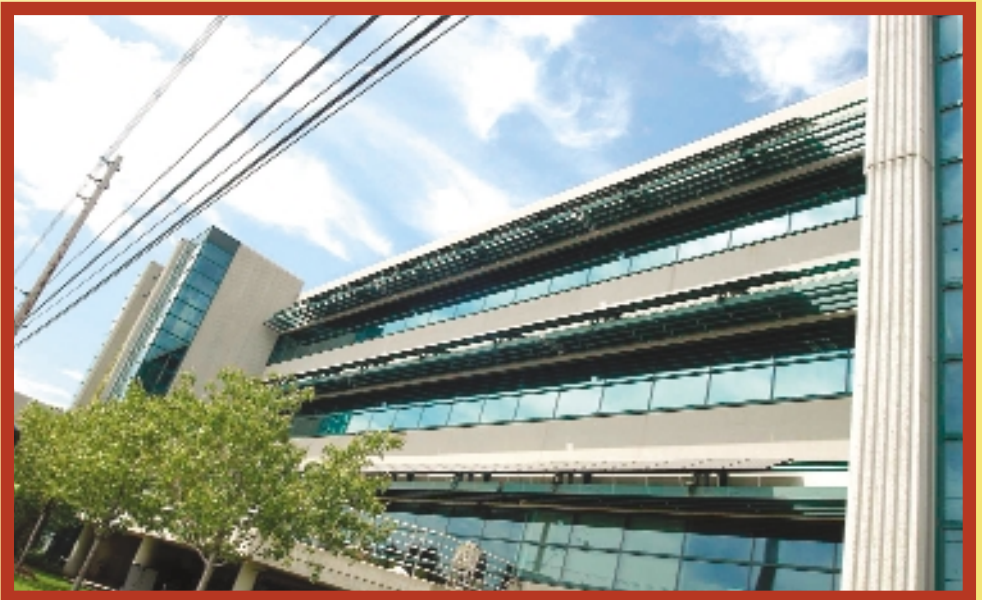
In 1996, during the original construction of Toronto Hydro's 500 Commissioner Street work centre, solar shades were added above all the windows. The purpose was to cut down on the sunlight and heat entering the building. The solar shade system was a perfect fit to installing a solar power generating system.
