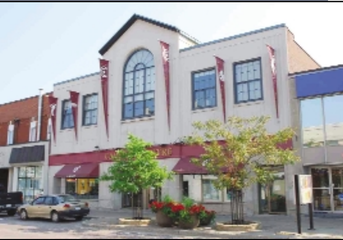
The Capitol Centre in downtown North Bay received financial incentives for their conservation and energy efficiency upgrades (photo courtesy of North Bay Hydro).
