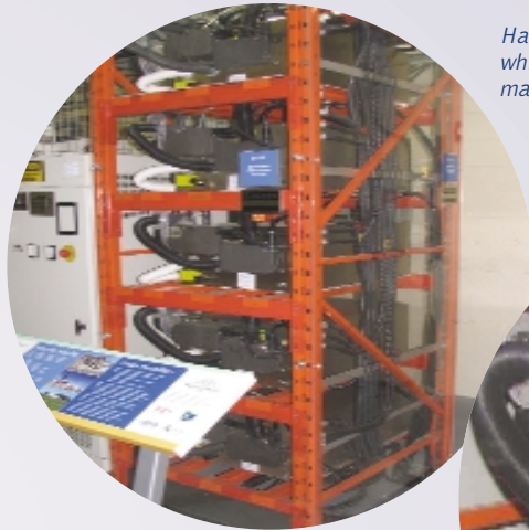
At the heart of 'The Electricity On-Demand' pilot project are ZEBRA batteries, which employ advanced sodium-nickel-chloride electrochemistry. (Photo courtesy of Halton Hills Hydro)
