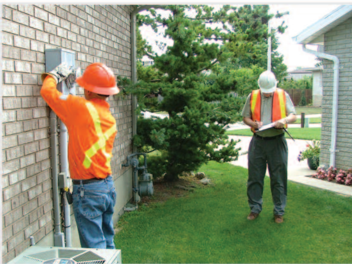
Smart meter deployment was carried out by C-K Hydro crews, who played a critical part in the initiative's success.
